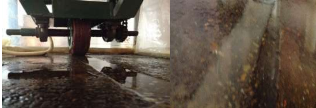
Figure 21: Rutting place on the pavement
