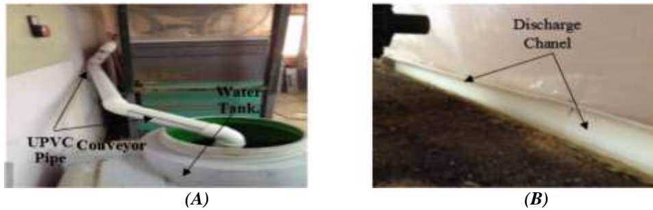
Figure 6: A) Conveyor Pipe, B) Discharge Channel.
