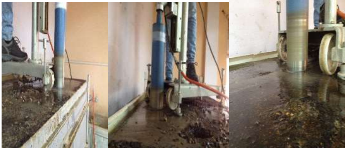
Figure 19: Cores extraction
